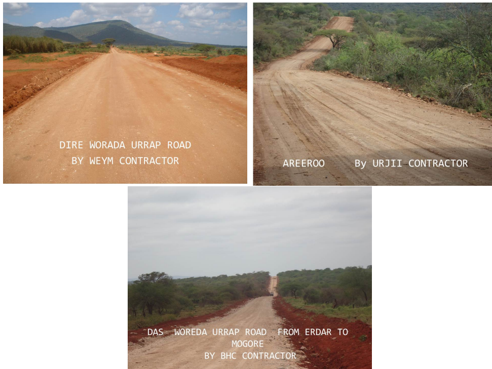
Figure 2: Completed URRAP roads (pictures are taken from Oromia Roads Authority).
